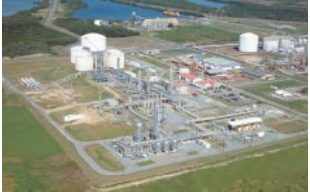
One of our larger gas processing plants
