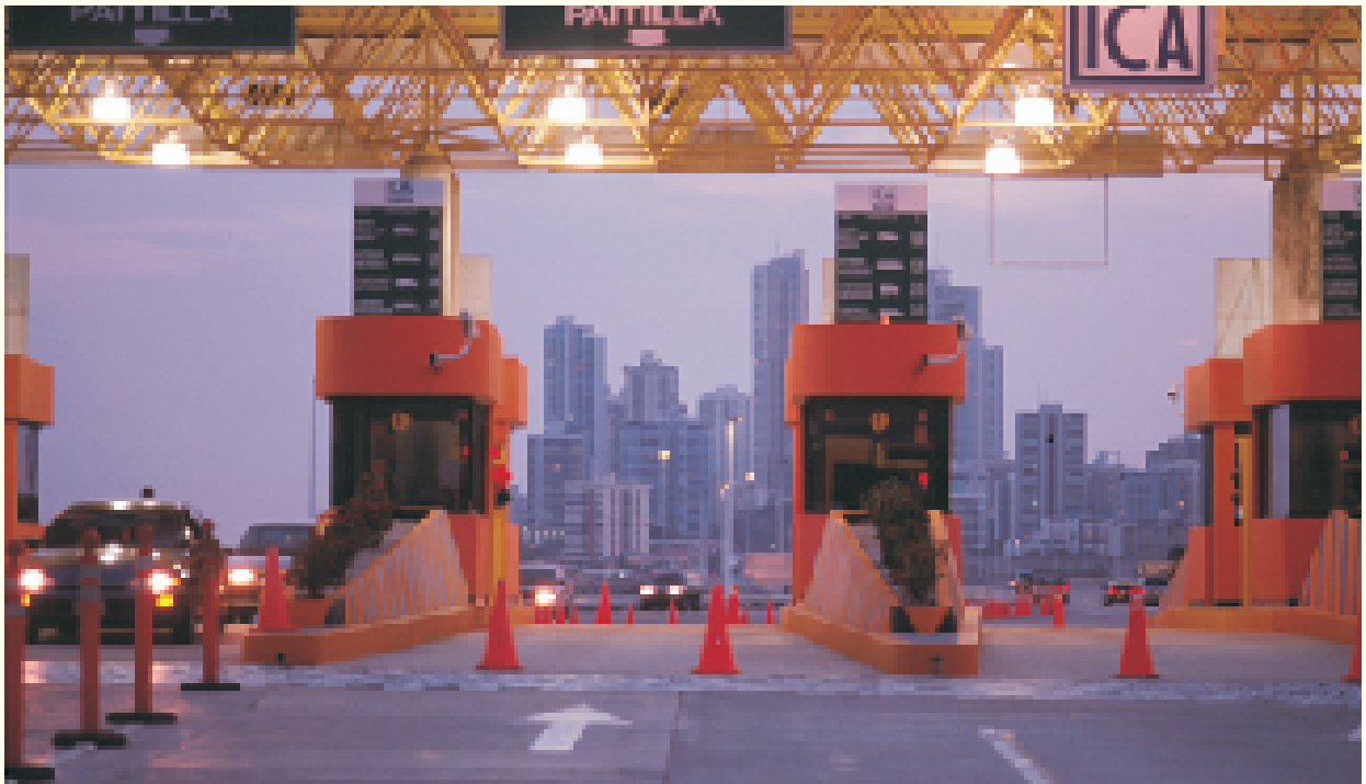
Toll Booth at the Southern Beltway (highway that connects the Tocumen International Airport to the City)
